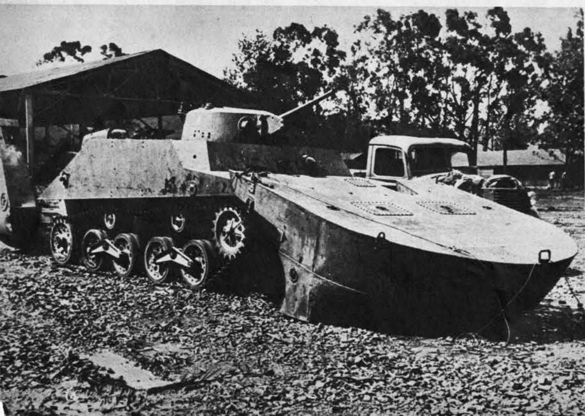
Jap armored oddity (above, below) is amphibian tank which "swims" with the aid of large barge-like pontoons fastened front & back. Pon-
